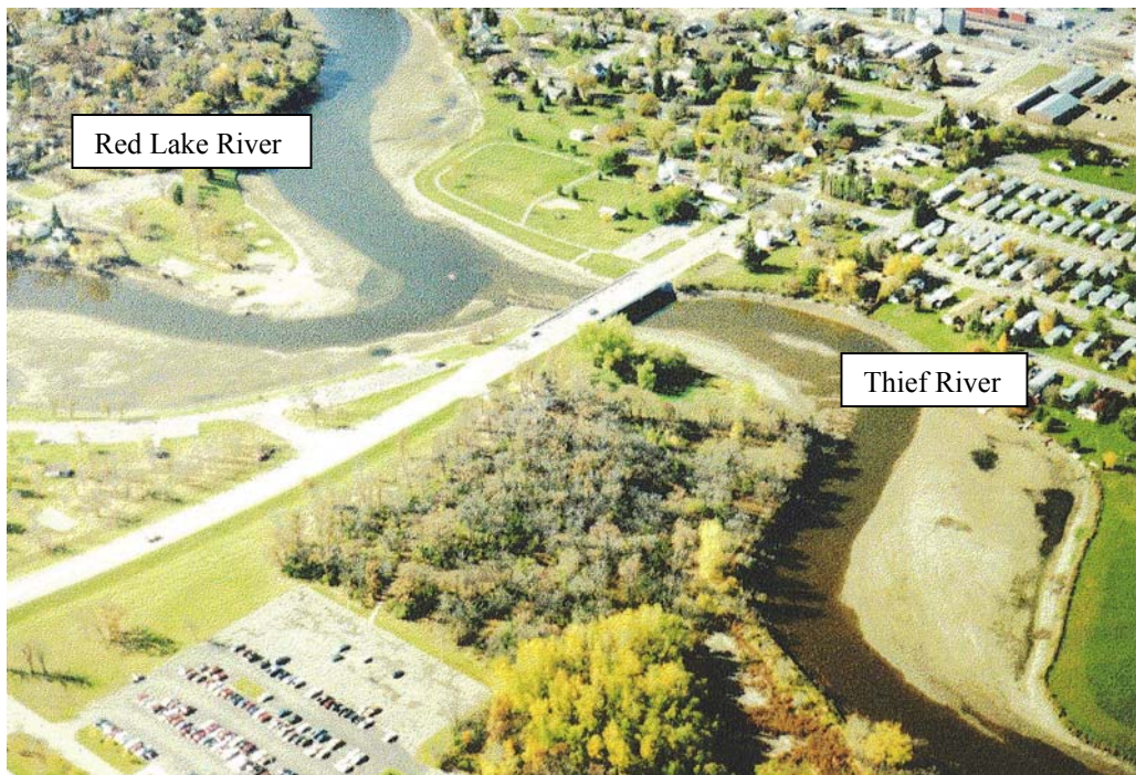
Figure 38. Aerial Photo of Thief River/Red Lake River Confluence.
